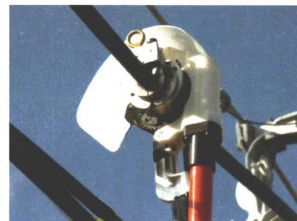
**STEP # 6.** Before the tool is placed on the conductor make sure the blade set ring is pushed all the way in. Turn the handle counter clockwise to open the tool, placing the tool on the conductor against the tool stop. While pushing the tool up slightly, seat the cable in the lower half of the jaw. Begin turning the handle clockwise closing the bushing around the cable until it is fully closed, an audible click will be heard.
