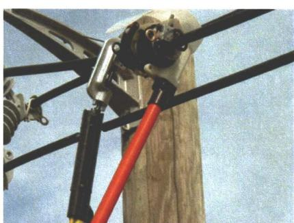
**SHORT-CUTTING THE TWO STEP OPERATION WILL RESULT IN DAMAGE TO THE TOOL. THE MID-SPAN PART OF THE BLADE IS NOT DESIGNED FOR 25 & 35 KV INSULATION REMOVAL IN ONE STEP.**
