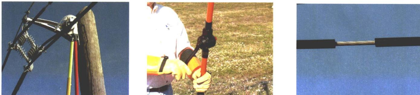
STEP # 10. Turn the handle counter clockwise to open the tool and remove the tool from the line. Using a grip all stick remove the MTS Tool Stop from the line. This concludes the stripping operation.
