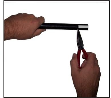
3. Peel scored semi-con segments with needle nose pliers or other suitable tool. Perfectly scored semi-con is cleanly removed without damage to underlying insulation.
