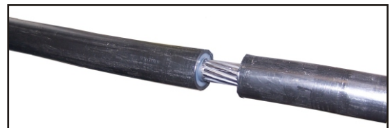
Fig 6: Step 10 - Completed strip.
